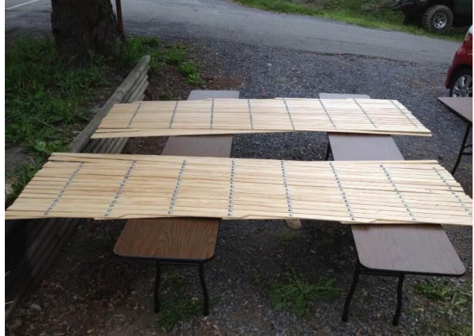
Figure 15 Two khana sections completed
