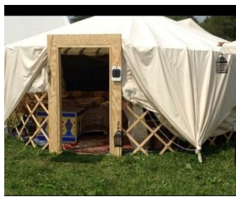
Figure 46 Canvas on and sideswalls pulled up
