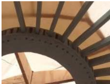
Figure 32 Toono ring with arches on top
