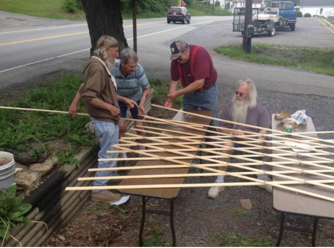
Figure 14 Bolting the strips together
